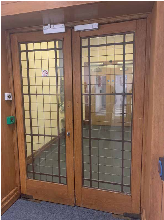
A heritage copperlight glazed door in tandem with a new certified fire doorset
