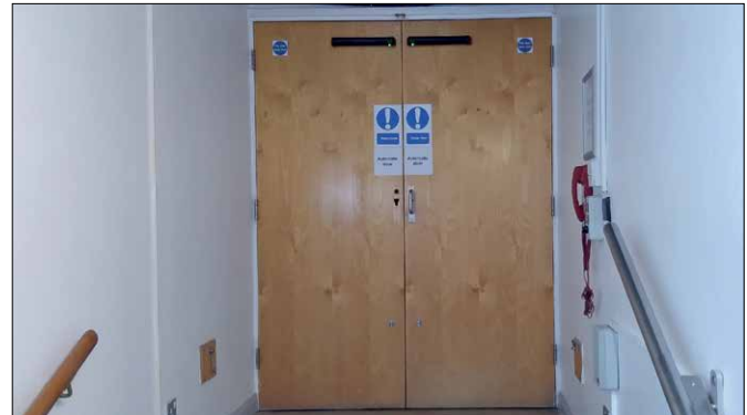
Electric locking devices installed on escape route doors need to suitably fail-safe.
