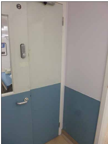
Fire doors with only two hinges need to be assessed in terms of what is suitable and sufficient.
