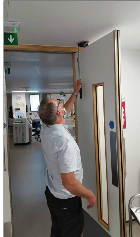
Checking the top edge of a door leaf during a Type 1 inspection
